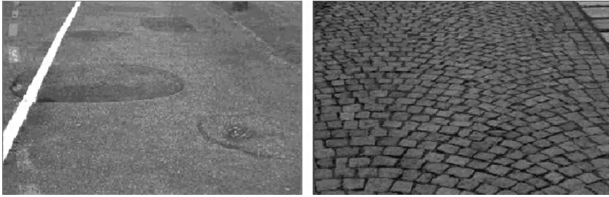
FIGURE 18.2. Typical defects of suburban and urban roads, relevant to vehicle comfort; at left a patched tarmac; at right a stone block pavement.
